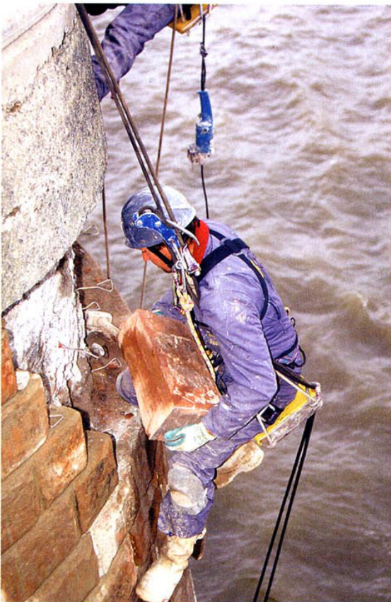
Figure 6: Rebuilding of the seawall
