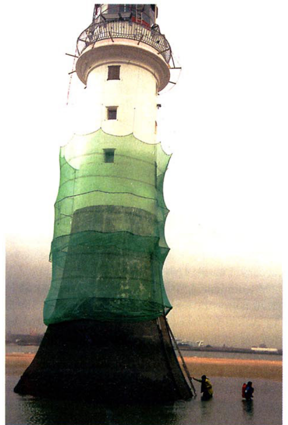
Figure 7: Containment net positioning
