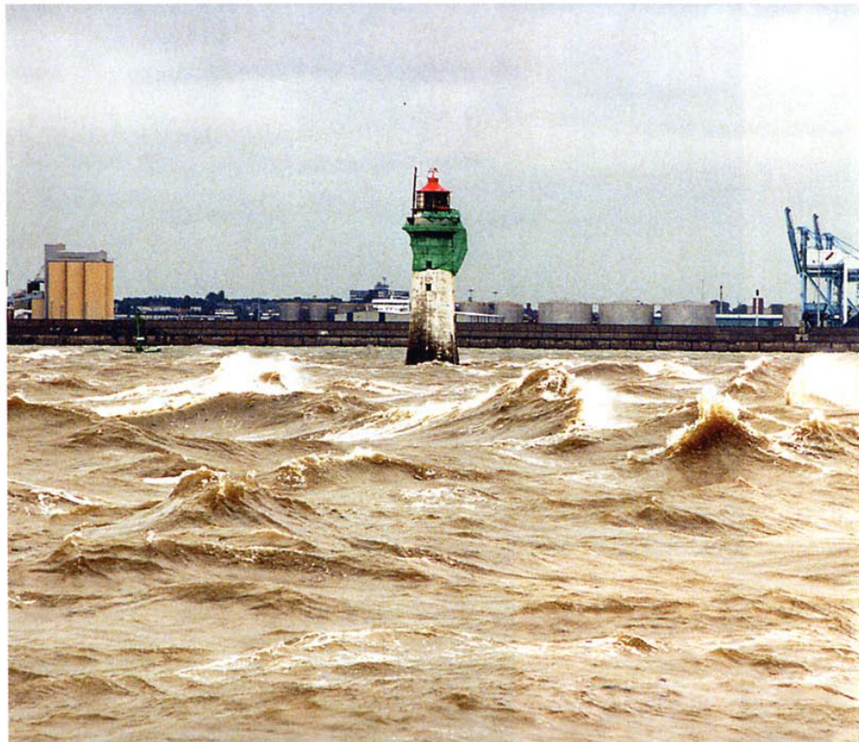
Figure 4: Project site at high tide
