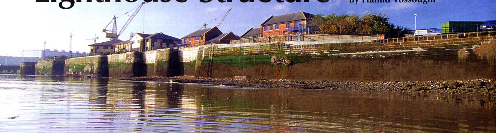
Figure 1: Priory Wharf seawall
